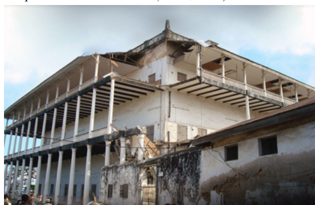
Figure 2. A corner section of the House of Wonders that collapsed in November 2012 (WMF, 2017)
