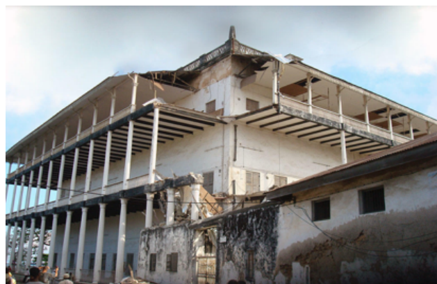
Figure 2. A corner section of the House of Wonders that collapsed in November 2012 (WFM, 2017)
